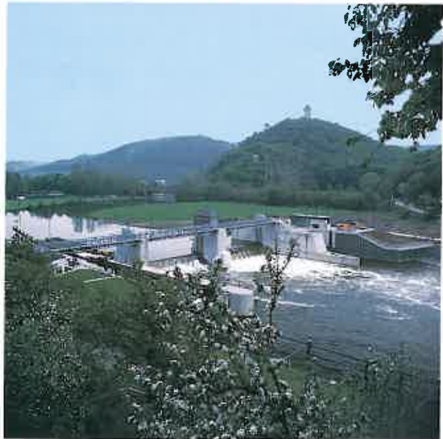
Nassau barrage weir on the R. Lahn
