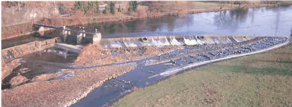
Weir on the R. Sieg with new fish ladder
