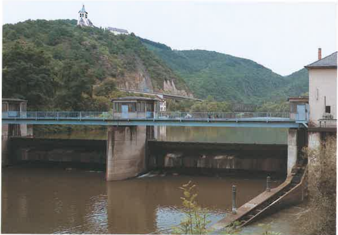
Lahnstein barrage weir with old fish ladder
