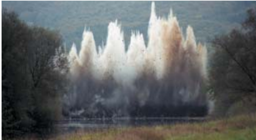
Blasting a weir in the loop of the R. Sauer in Luxemburg with aids from Rhineland-Palatinate
