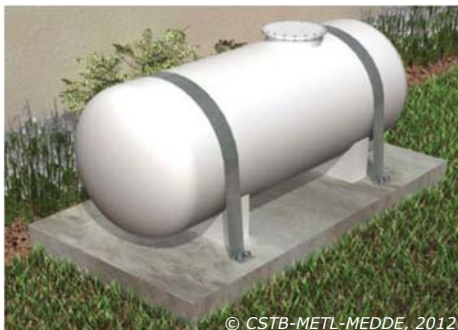
Example of anchoring an oil tank
