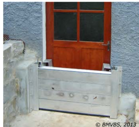
Examples of "flood-adapted construction (I.3.1)" (left) and "flood-proofing property (I.3.2)" (right) (cf. http://www.bmub.bund.de , Hochwasserschutzfibel (= Flood Protection Handbook))
